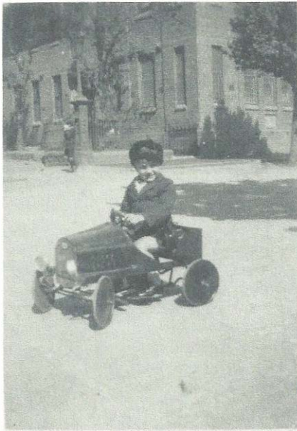
COLLIS MOSS OPPOSITE ST MARKS CHURCH LIBRARY
